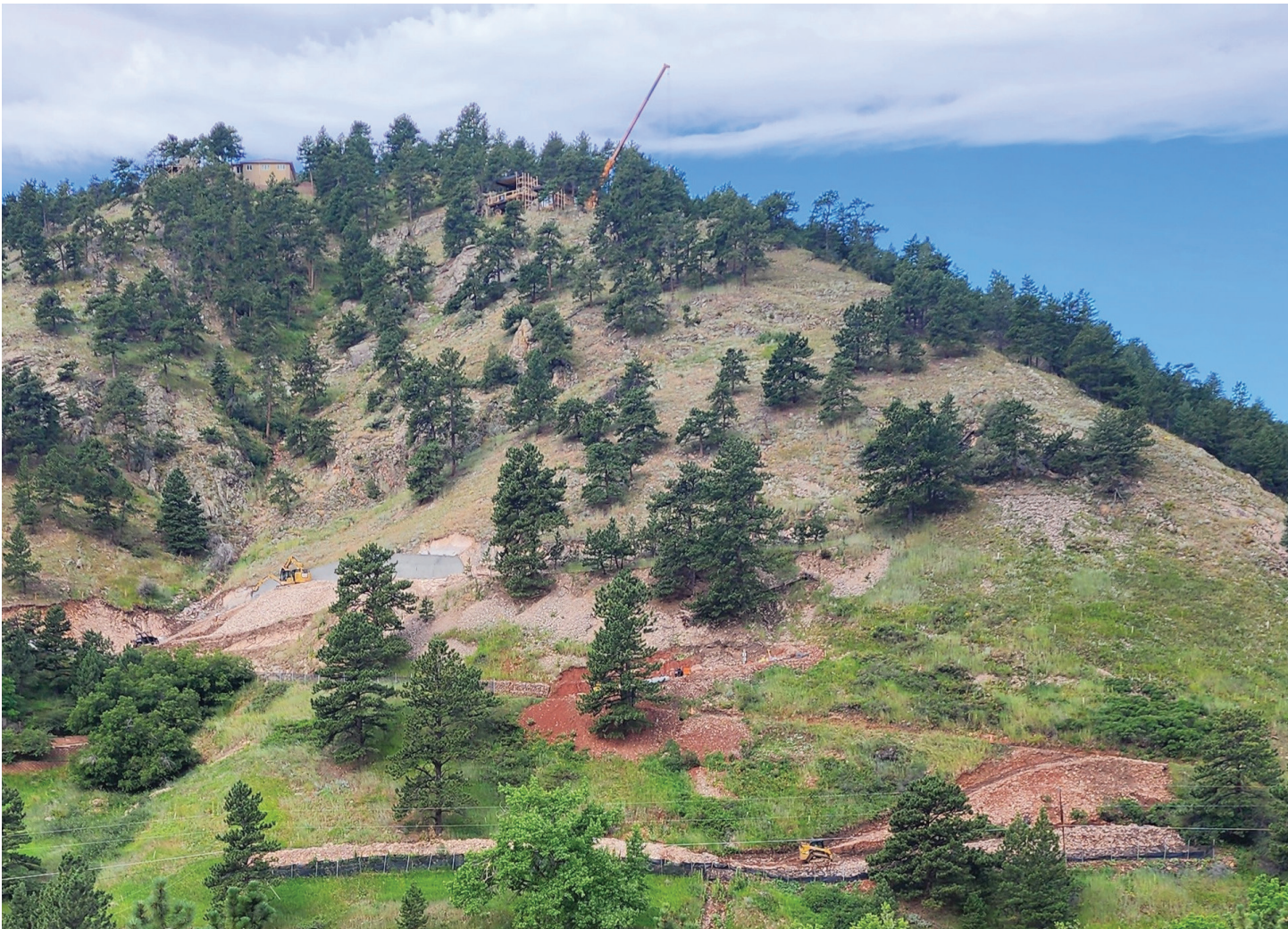
Construction Photo by Mark Johnson
