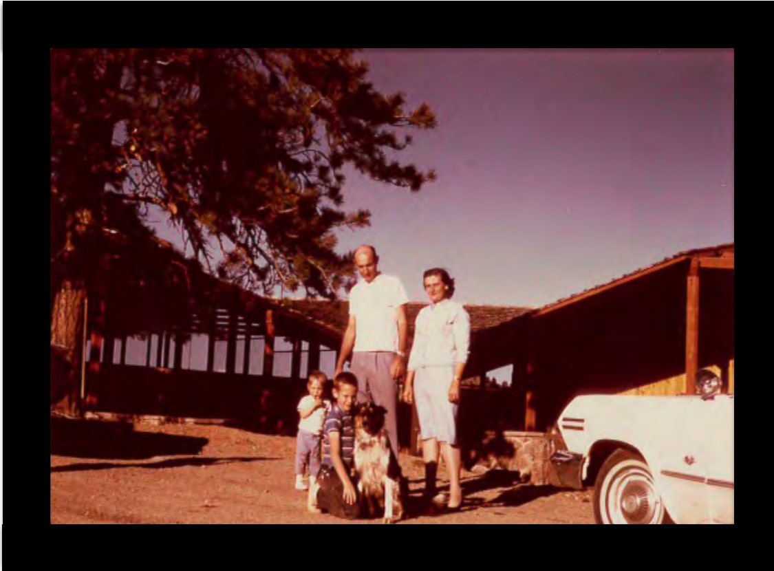
Joe Erni with wife Betty, Nancy and Ken at their new home construction on Timber Lane in 1961
