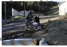
constructed a wood timber retaining north of the building entry to prevent erosion onto the new paved area
