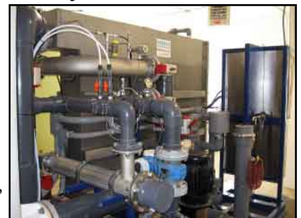
The new filtration plant.
