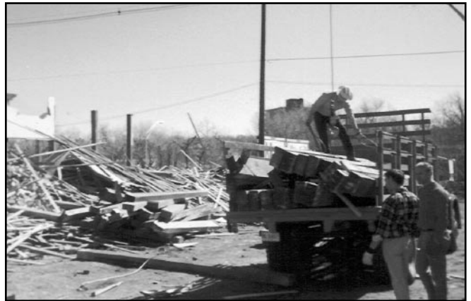
Salvaging lumber for the firehouse from a building blown down by wind. John Seward is on the right.
