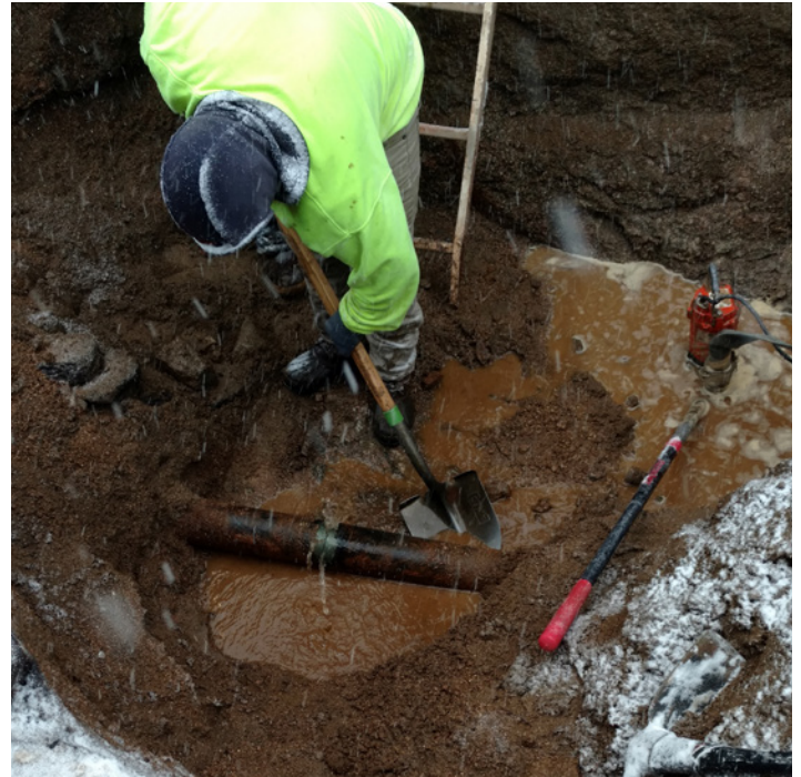
PBH Water Department crew working on the Wild Horse Circle water main break in January.
