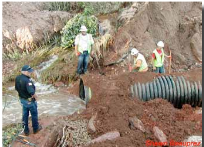
Bob, on left, at North Cedar Brook Reconstruction.
